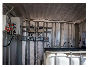
The Chemical Dosing Unit Plus (CDU+) is a pH and turbidity correction system used to treat extracted groundwater with a high or low pH, high turbidity and Total Titratable Acid (TTA) levels. It does this by adding calibrated amounts of pH modifiers (acids/bases) and flocculants/coagulants to the effluent stream. When used in conjunction with a clarifier, it is also highly adept at dealing with turbid, site surface water runoff volumes, prior to them reaching stormwater systems and waterways.
